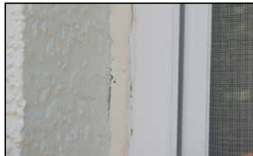
Sealant adhesion failure
