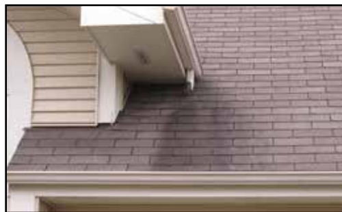
Downspout discharge directly onto shingles
