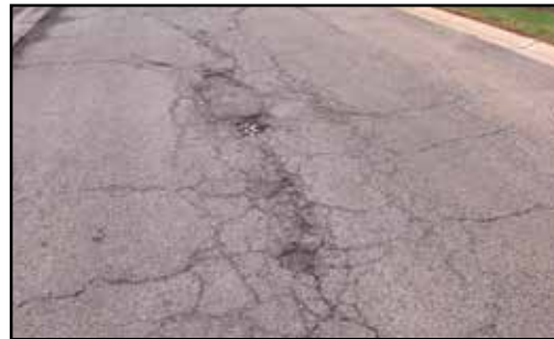
Cracks and potholes
