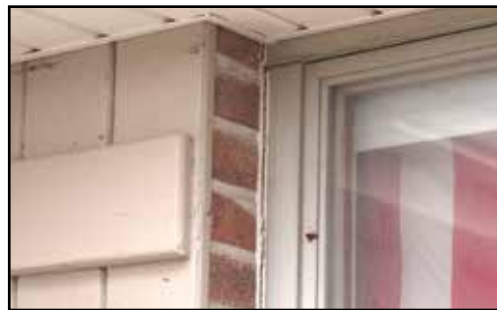
Sealant deterioration
