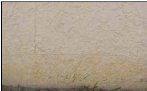
Crack at side elevation
